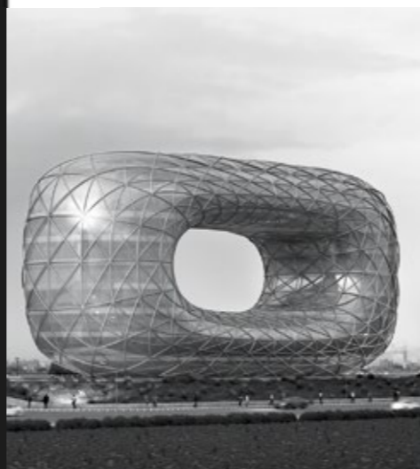
Multifunfional building Shangai - China Works in progress
